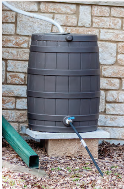
Rain barrels capture and store stormwater for uses such as watering gardens or filling up wash buckets
